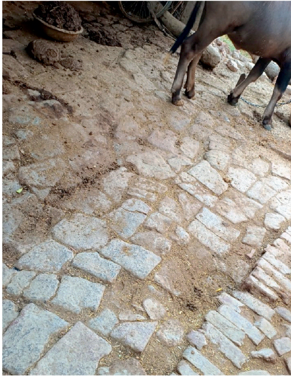
Fig. 20: Ancient bricks used for the construction of animal enclosures
